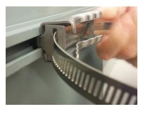
**Step 2**Feed the banding through the saddle and out of the other side, creating a loop
